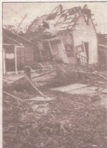
DESTRUCTION: A resident survived Hurricane Andrew in Cauley
